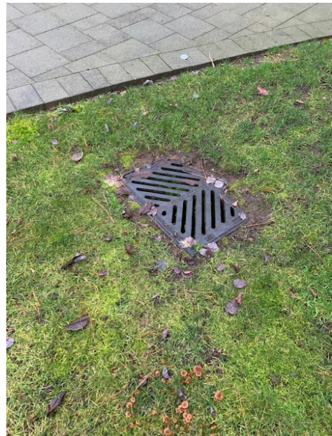
SE 27 th St. South Edge Catch Basin – Point D
