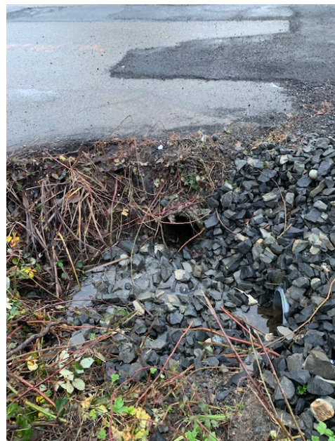
End of open channel – Culvert entrance Point G
