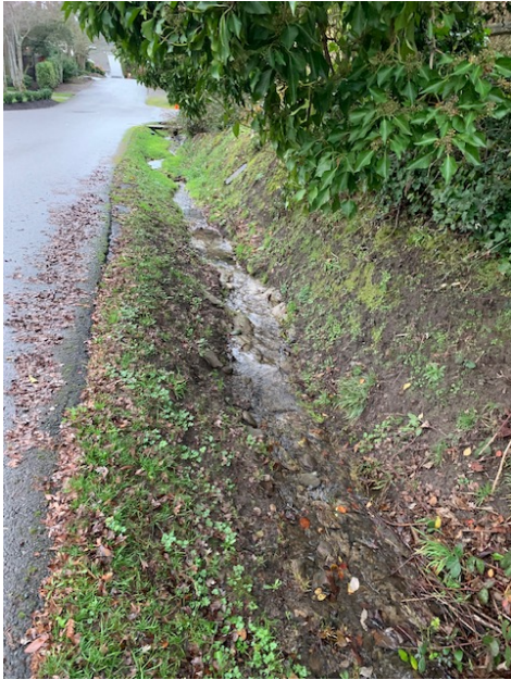
Open Ditch Across the site - Looking Downstream
